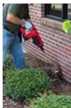
Angle beneath slab
