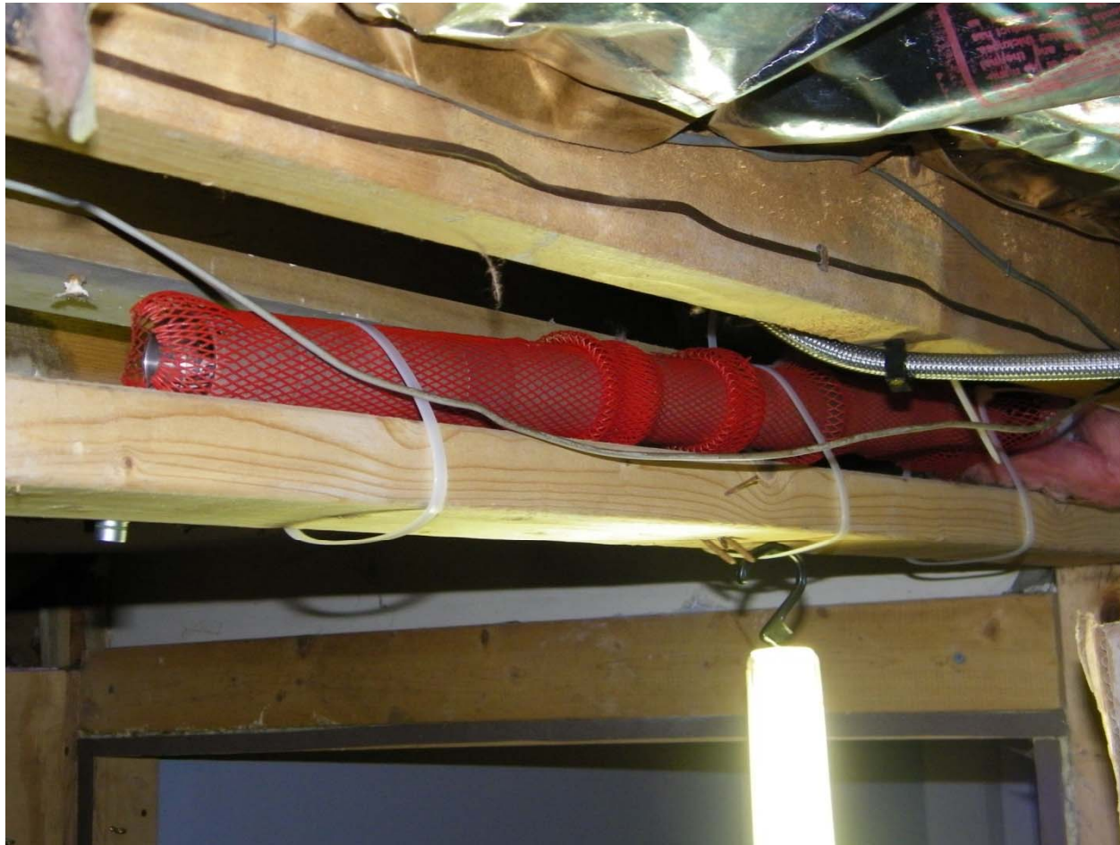
View of Ion Science GasClam installed near entrance door to cellar.
