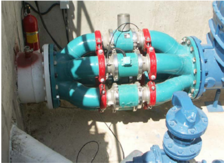
Figure 4. RAVEN-PROTECT valve system installed at the exit of a drinking water storage tank
