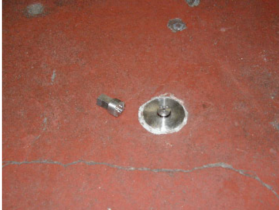
Farallon VOC Monitoring probe with cap partially installed. Also shown is cap installation tool.
